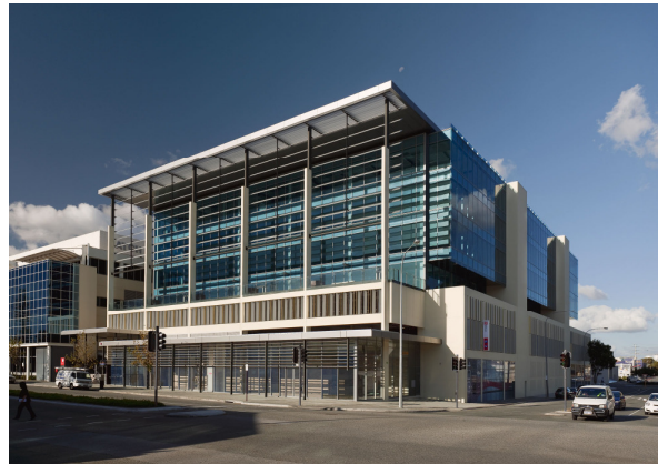
One30 Stirling Street: the new home for HLB Mann Judd from mid-January 2010, with its key balcony feature, overlooking Stirling Street and the city beyond
